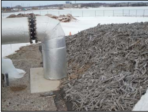
BIOFILTER SYSTEM (Tree Roots)
